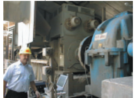
in copper mills
